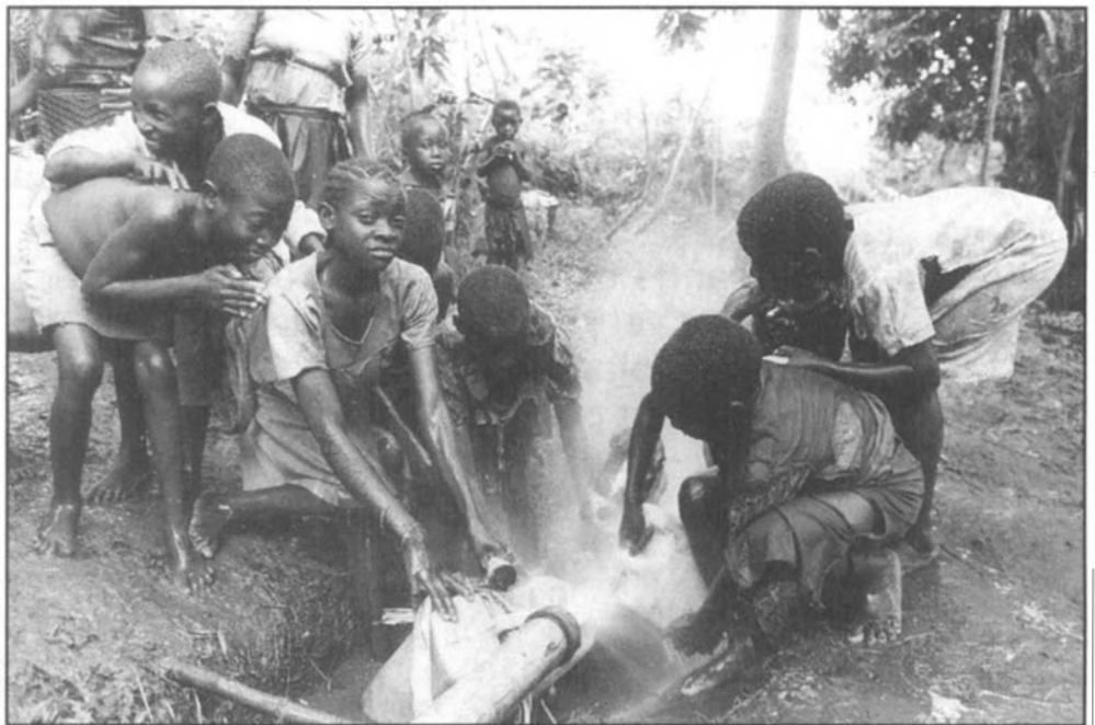
A water-pipe in the Ruentores mountains of Uganda's Bwera District: the local communities have no control over water pressure.
