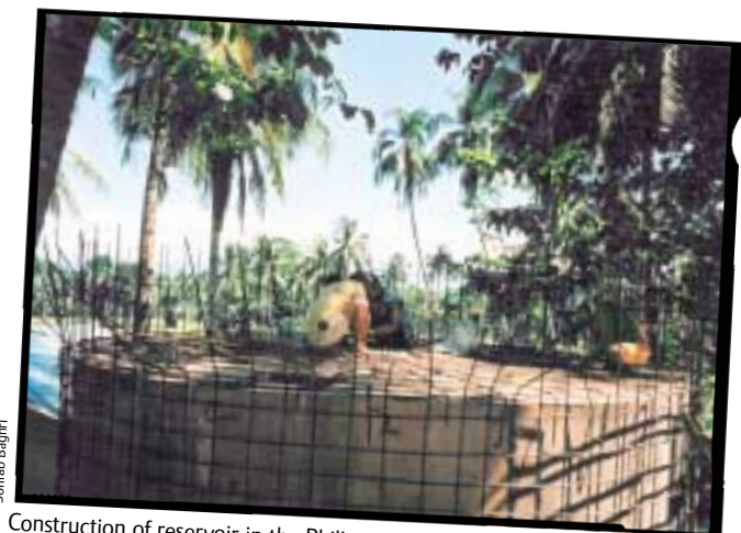
Construction of reservoir in the Philippines
