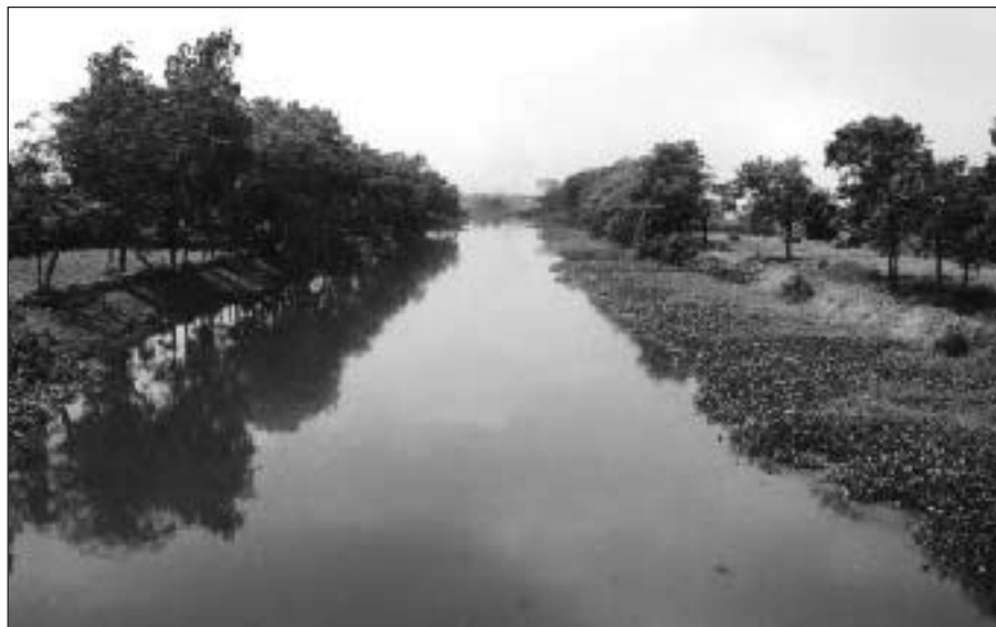
Untreated wastewater is pumped from Kolkata via a series of secondary canals like this one to several hundred fishponds
