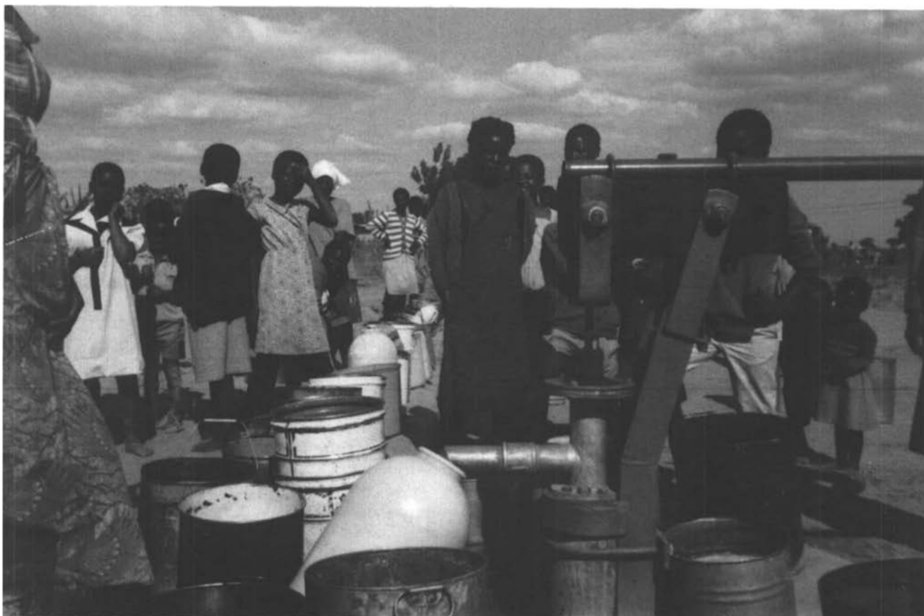
Heavy use may account for the greater number of breakdowns of Bush Pumps.
