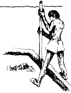
Municipal worker cleaning small open drain
