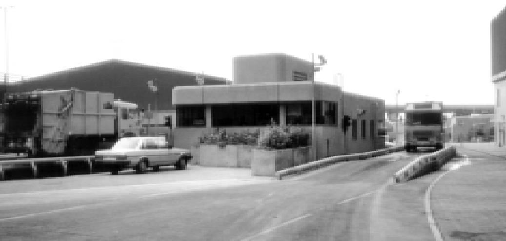
Photo 1.1 The entrance to a private sector transfer station in Hong Kong
