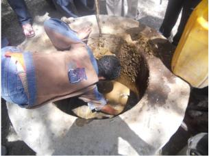
Figure 4.3. Mixing slurry by hand at the inlet of a biogas digester in a rural household near Debre Zeit
