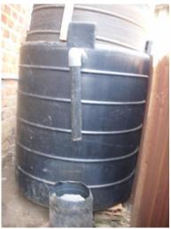
Figure 3.1. Floating drum digester in Kajansi
