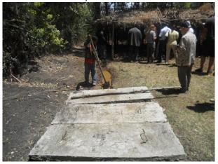
Figure 4.4. Shallow channel taking biogas digester outflow to compost heaps at a rural household near Debre Zeit
