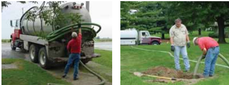
Figure 5. Emptying of the Septic Tank
