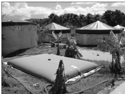
'Oxfam tanks' of 95 and 70 m 3 capacity being utilized in Gonaives, Haiti
