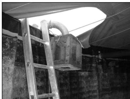
A wire mesh cage is fixed onto the tank inlet to aid in alum dissolution.
