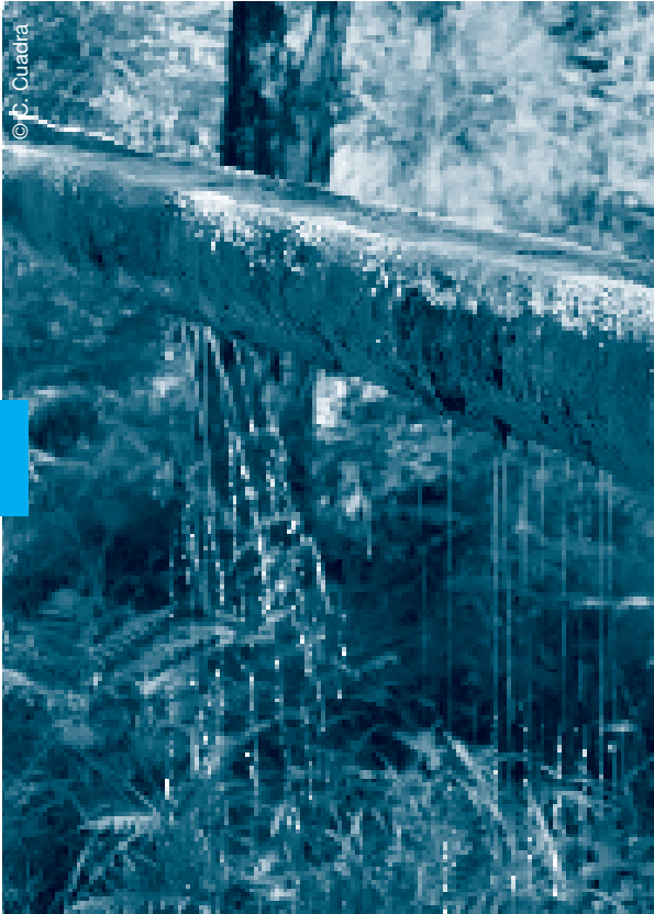
The traditional way of carrying water in 'pipes' made from tree trunks is far from efficient (Segura de la Sierra, Spain).
