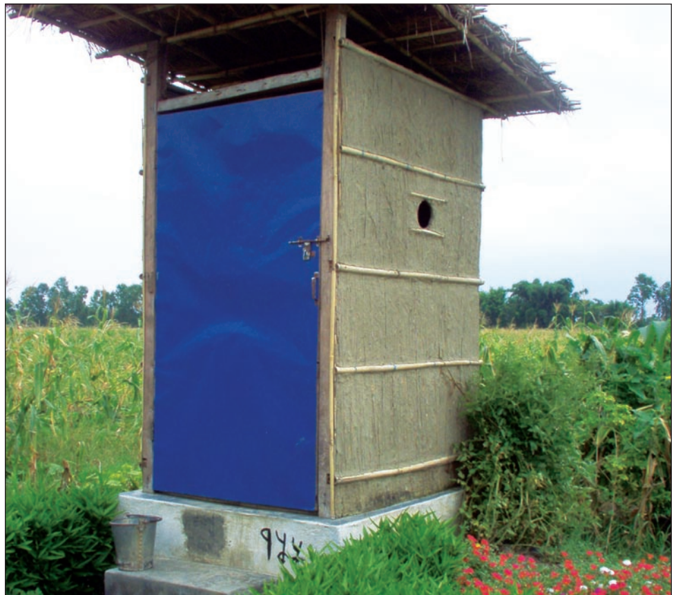
Community latrine installed after the SLTS programme intervention.
