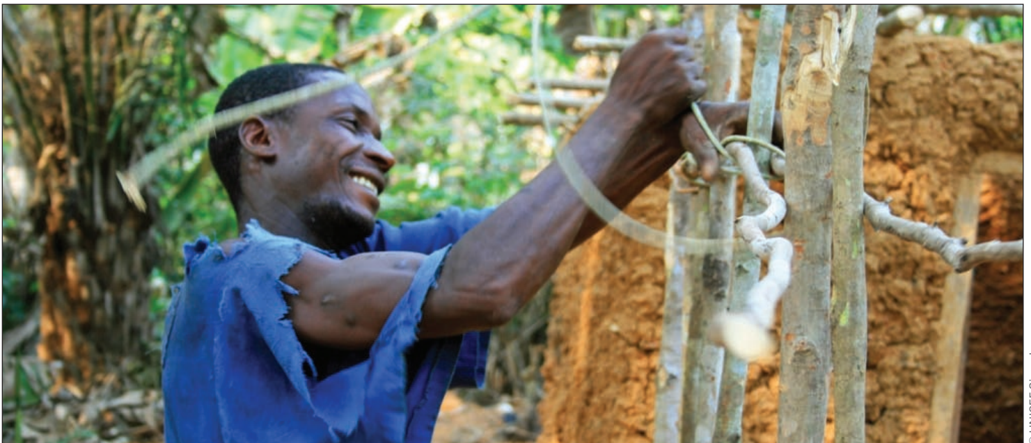
Community member building latrine from local materials.
