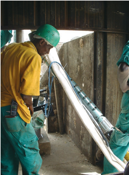
A private operator installing a water pump
