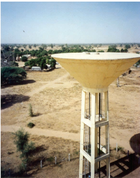
The Refane water tower in Senegal
