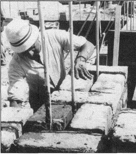
Bamboo poles reinforce the adobe walls.
