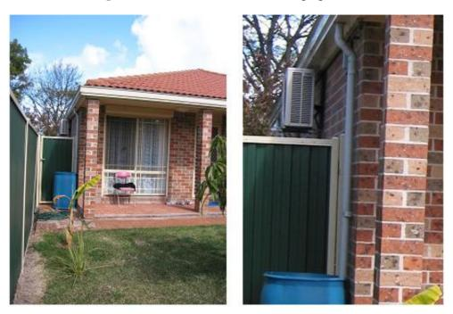
Figure 7. User modification to storage gutters.
