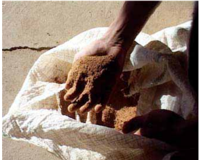
Six pounds (2.7 kg) of sawdust are mixed with 60 pounds of good quality clay
