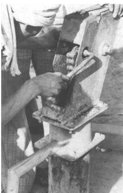
Good system design includes a maintenance programme.
