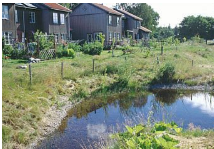
Figure 1: Ecovillage Understenshöjden, Sweden - one of the project sites
