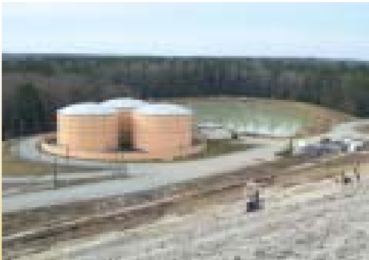
An expanded leachate containment system using glass-lined steel tanks. Each tank has 330,000 gallon (about 1.3 mega litres) capacity. In the foreground are landfill gas headers, connected to landfill gas wells, in a closed landfill cell. Jones Cross Roads Landfill Site, Delaware, USA.
