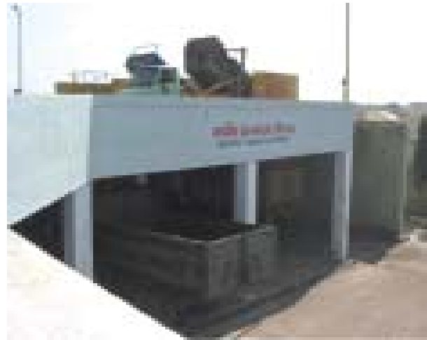
Transfer station, Rajkot city, Gujarat, India. Small vehicles climb a ramp to empty waste into larger vehicles stationed at a lower level. Transfer stations enable costs of transportation over longer distances to be optimised.
