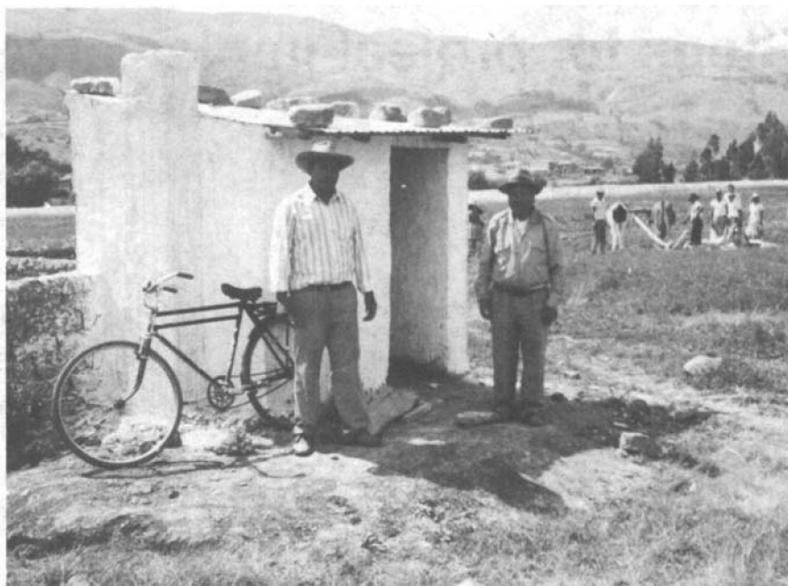
The project requires all participating families to construct latrines, most of which are a pour-flush water-seal design.
