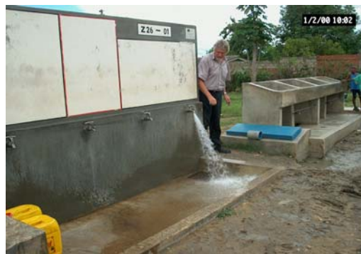
Figure 3-3: An improved communal standpipe constructed by JICA in George in Lusaka
