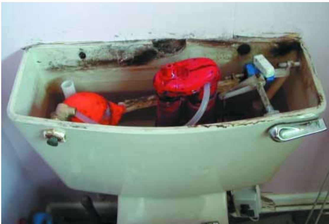
Plate 2: The Mecon Interrupter Device
