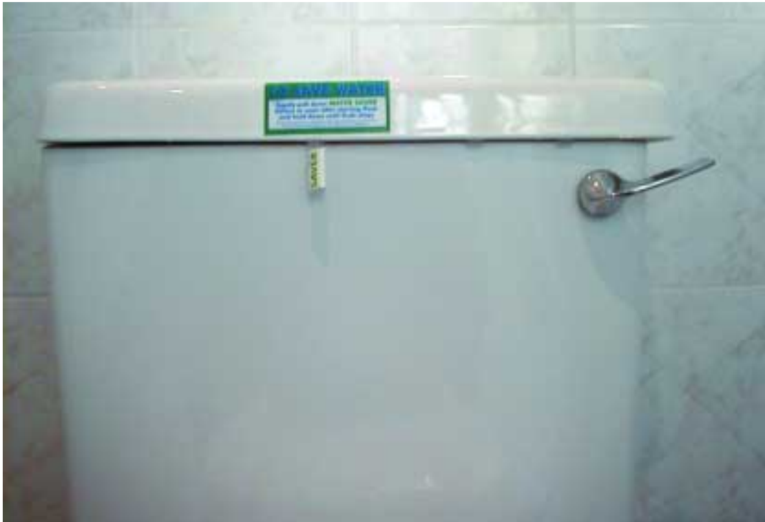
Plate 1: The Mecon high/low default Flush Device
