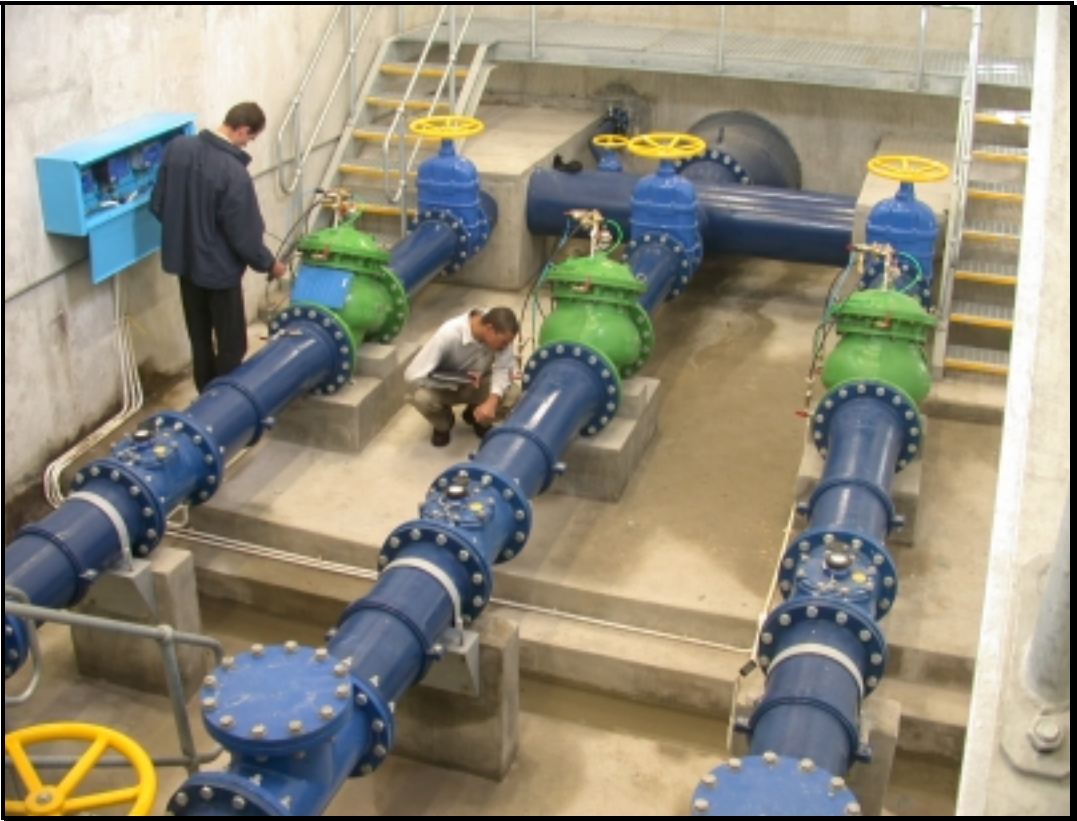
Figure 6: Internal View of a Portion of the 1065 mm diameter Chamber
