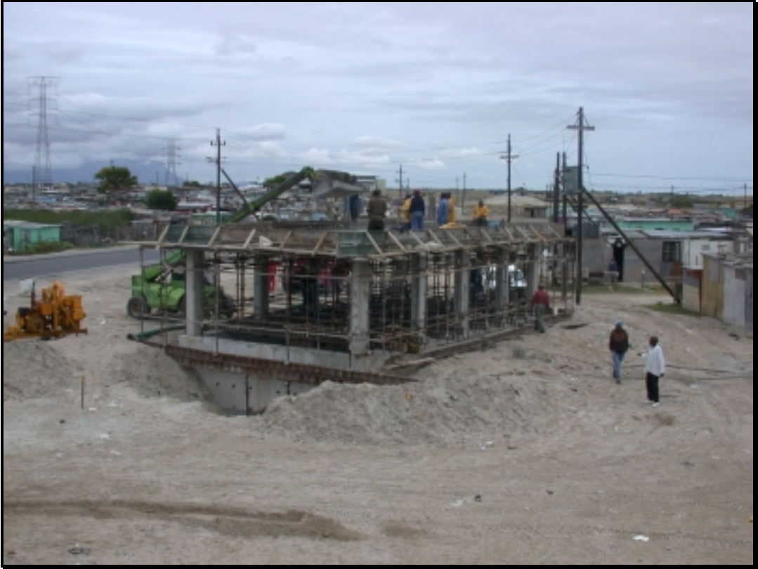
Figure 5: Partial construction of the 1065 mm diameter Chamber
