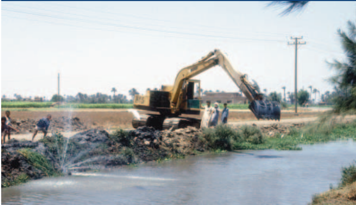
Plate 13 Dredging irrigation canal (Egypt)
