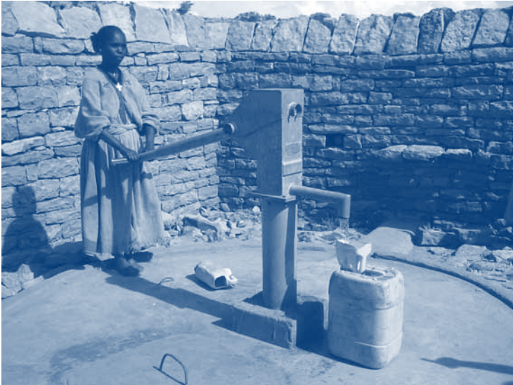
Figure 2.2. Laundry basin (top) and storage of filtered water with handpump (bottom) as part of a multiple-use system in Adidaero in Ethiopia (photos: Michiko Ebato)
