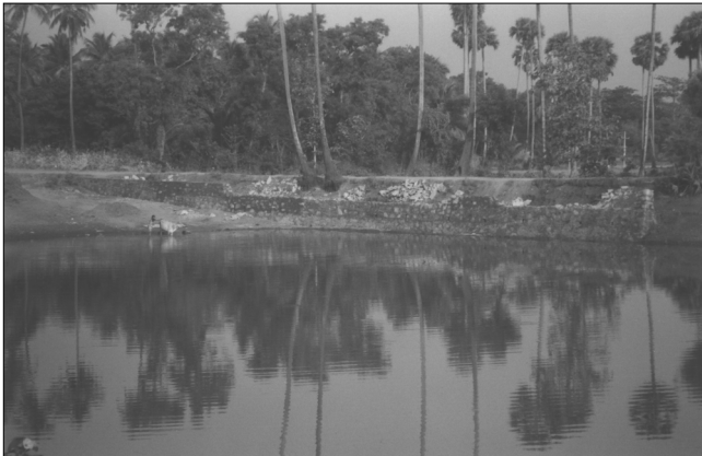
PHOTO 4.1 Side Protection work in progress
