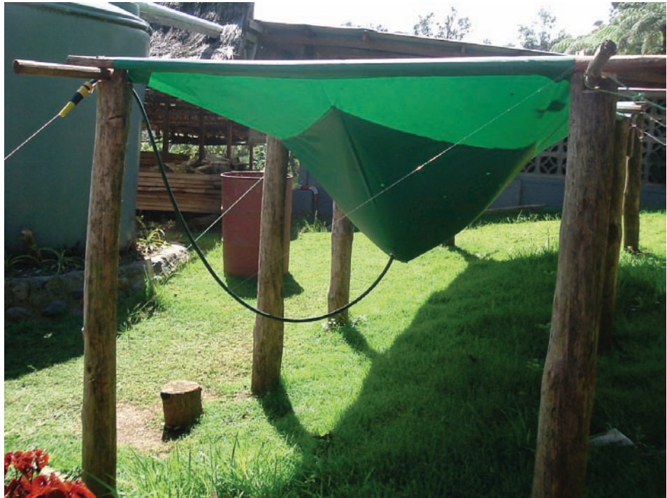
Figure 7 The portable water catchment enables households to have their own nearby water supply ATprojects
