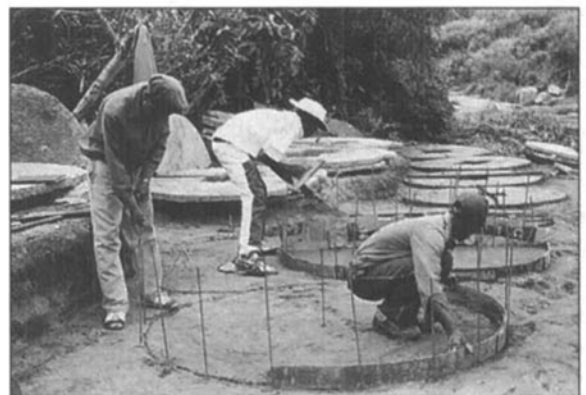
Constructing lids for the 5000-litre capacity tanks.
