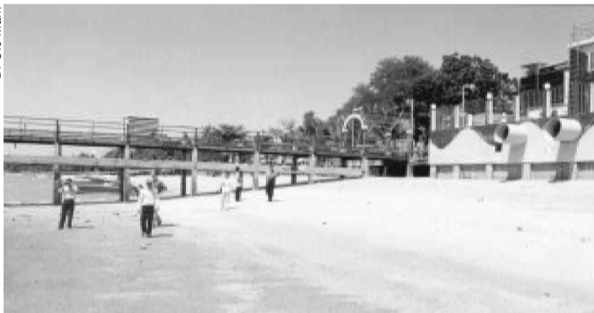
On the right, the combined sewer overflow discharges wastewater onto the beach after heavy rainfall
