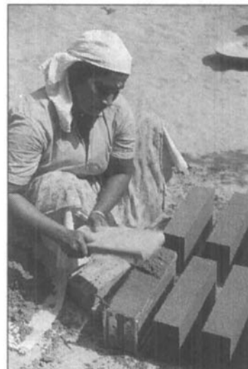
Preparing hand-made, solid bricks for latrine construction.
