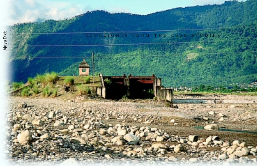
In the early 1960s the Tinau River in Nepal bypassed a recently completed irrigation barrage. The river embodies physical, hydrological, social, cultural and political variability. Total understanding is an unachievable goal.
