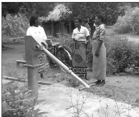
Many handpumps were failing not because of water scarcity but because of hardware breakdown (photo credit: WEDC/Peter Harvey)
