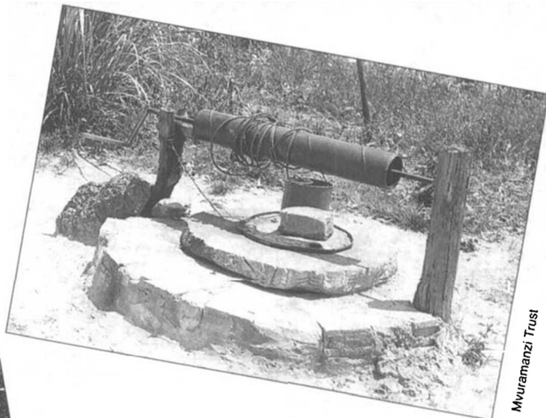
A fairly typical, traditionally upgraded well with raised lining, concrete cover slab, windlass and tin lid (above). An early upgraded family well (left). These wooden poles were replaced by more permanent brick columns.
