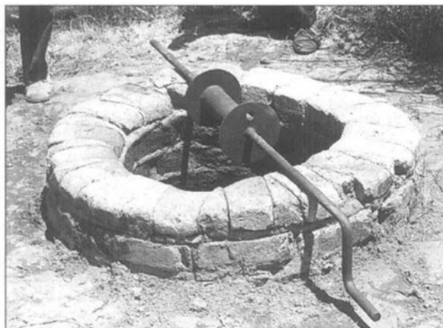
An old brick-lined well. The new windlass which will be used to upgrade it is being tested for size.
