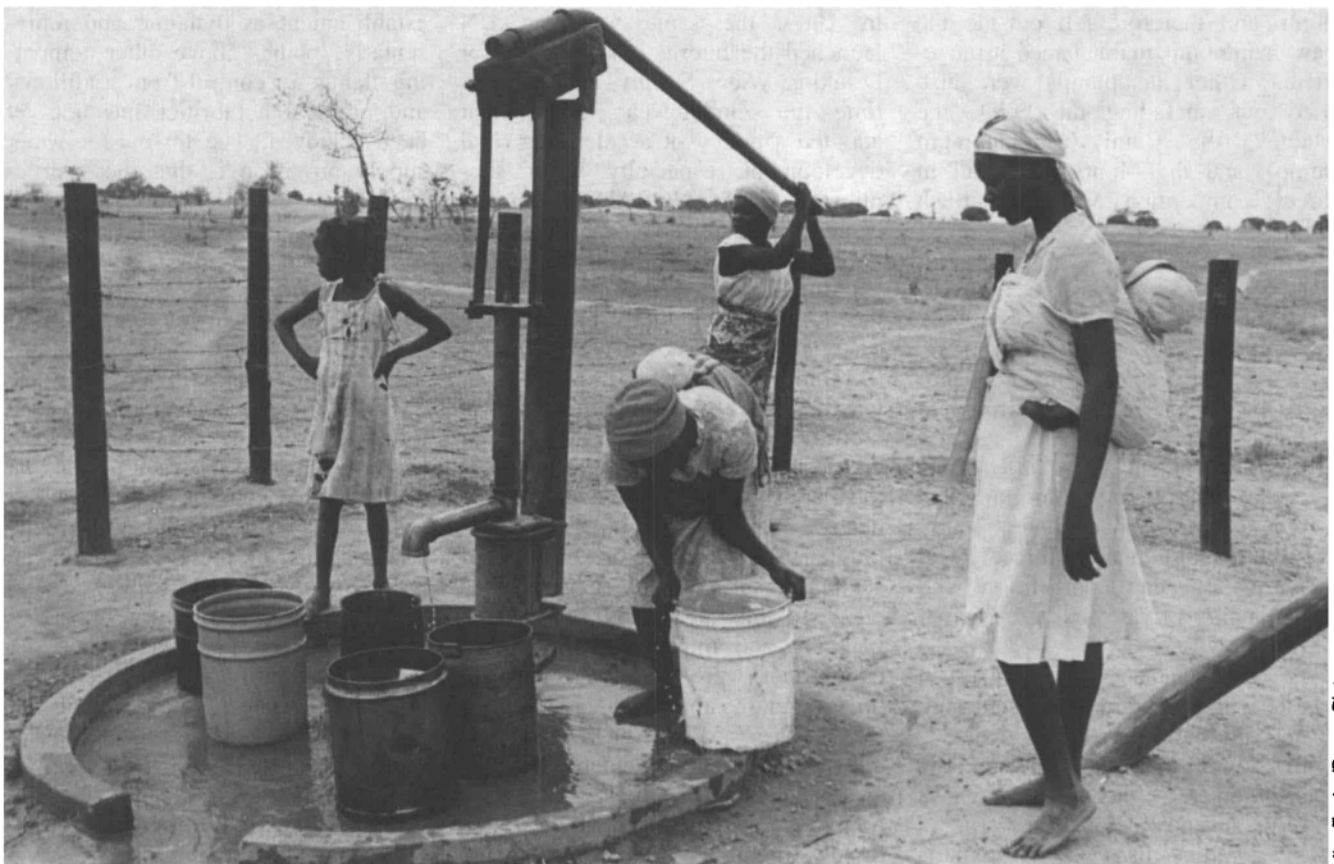
As the Bush pump was not patented, a family of Bush pumps was created, with the main common characteristic being the use of hardwood as a bearing block.
