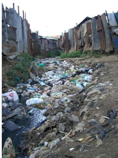
Figure 10: Blocked wastewater drains in Kibera, Nairobi
