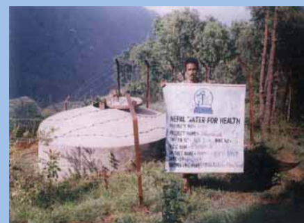
Reservoir tank (RVT) in Bhumlusalle (PN 1457z)
