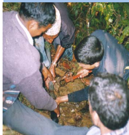
Fixing broken pipe line, Purna Dihi (PN 21b)
