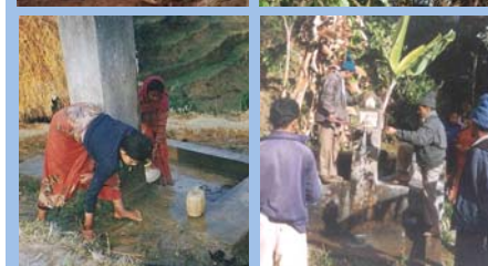
Maintenance work being undertaken in various projects
