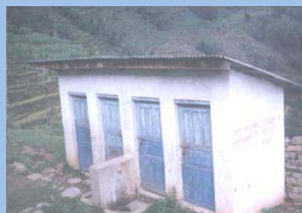
School latrines in Kharmi (PN 1766z)
