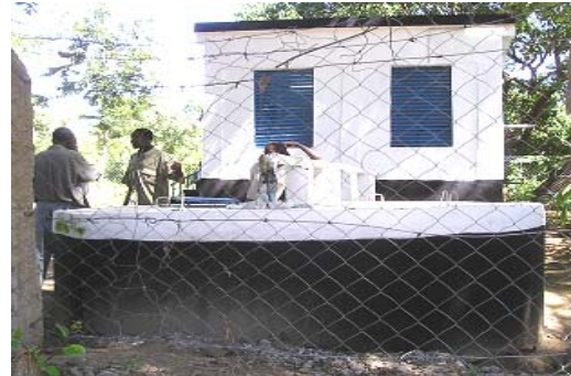
The completed well head with the pipe from the well to the pump.
