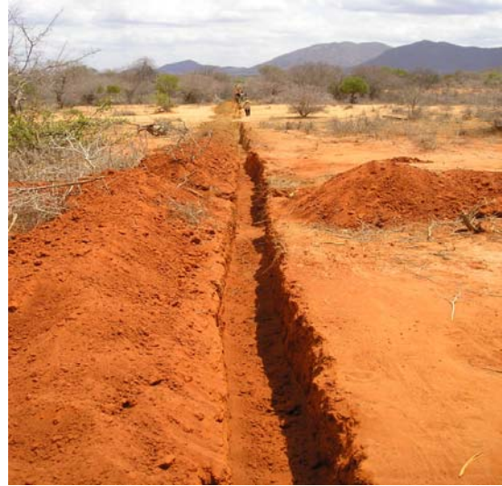
A trench excavated for laying pipes.
