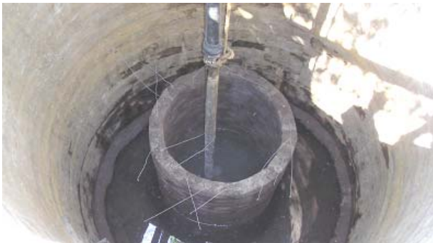
The small well shaft being sunk inside the wide diameter well shaft in the riverbank
