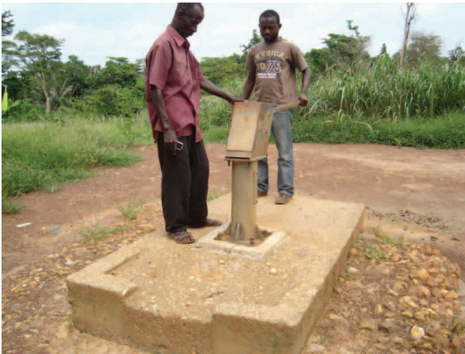
Plate 1: Abandoned rural water point-system
