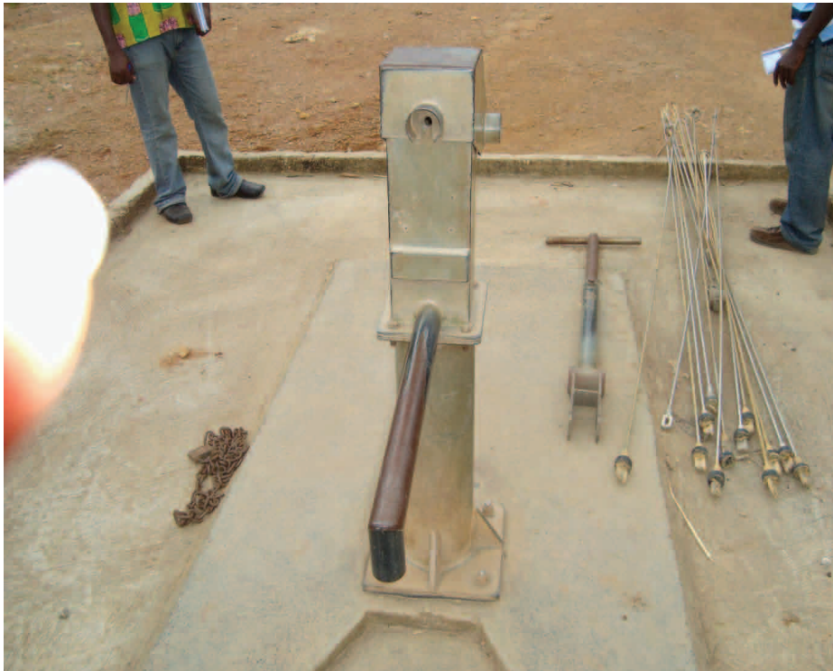
Plate 2: A typical rural water point-system under repairs
