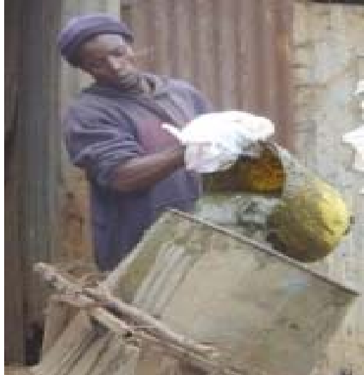
Picture 4: Manual way of emptying human waste from a pit latrine
