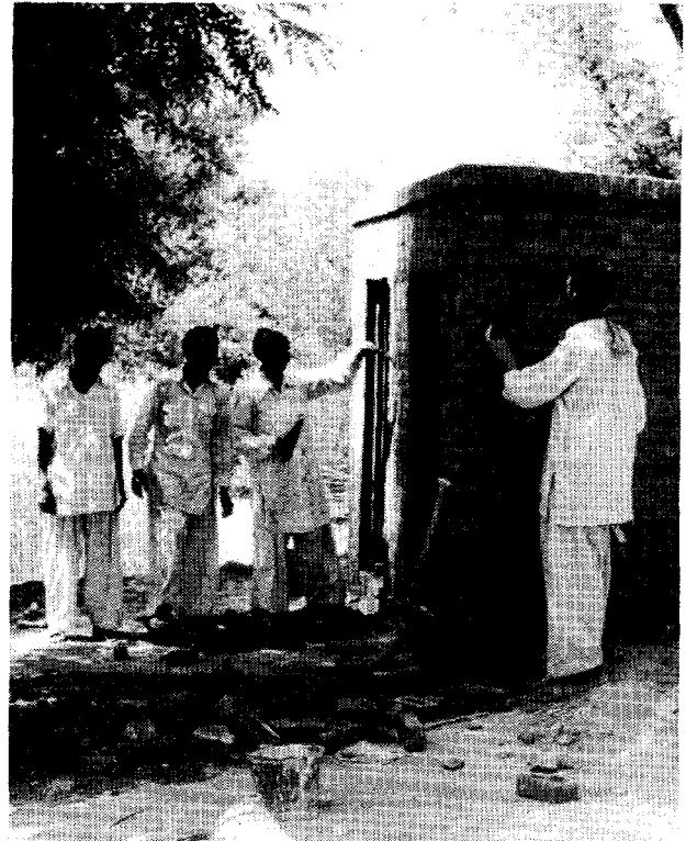
Village masons were trained and latrines constructed - including latrines for schools.
