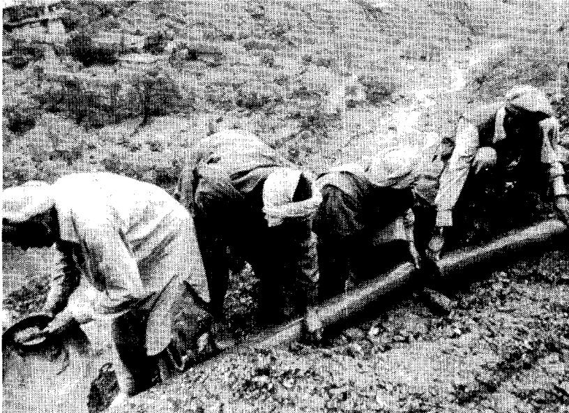
Maintenance of the gravity-fed system is carried out by the villagers who built the scheme.
