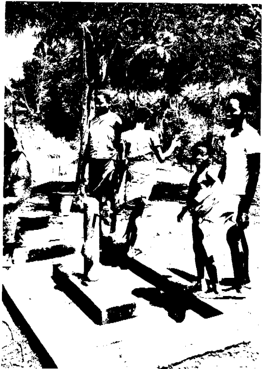
Photograph 16. Support is higher than top of tap. (Ghana)
