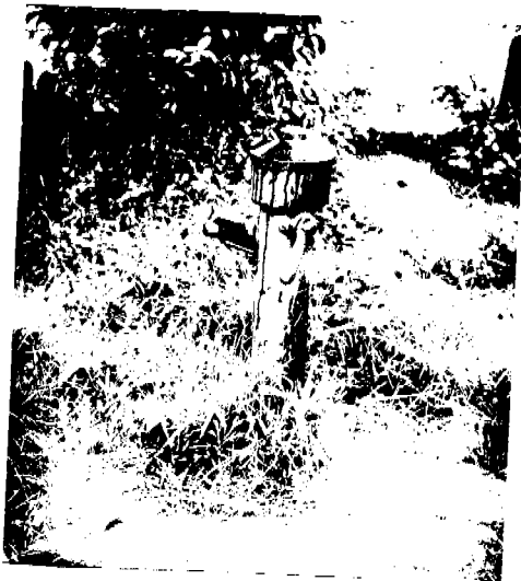
Photograph 4. Springloaded tap in cast-iron supporting construction (Suriname)
