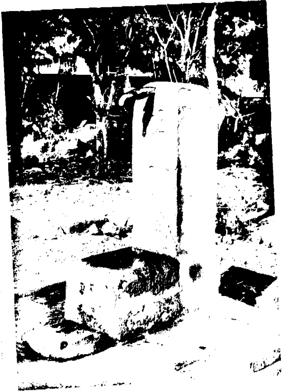
Photograph 17. Tap and piping supported by concrete pipe. (the top of the tap is higher than support) (Mauritius)
