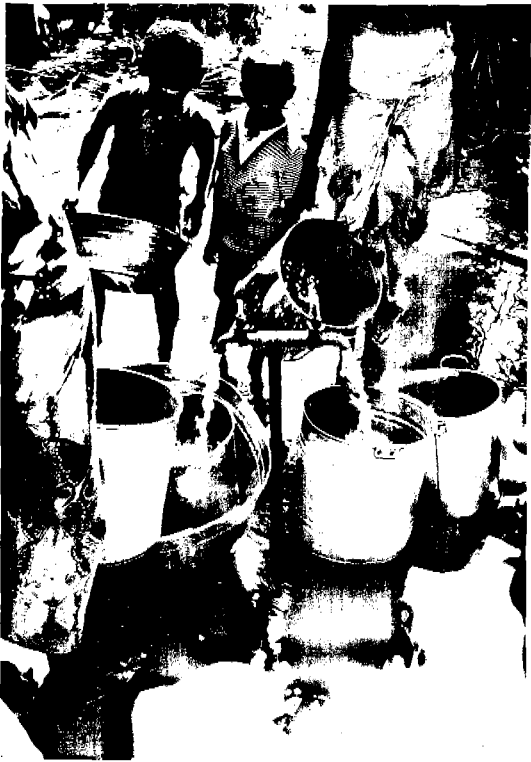
Photograph 15. Unsupported hydrant with two taps. (Zambia)
