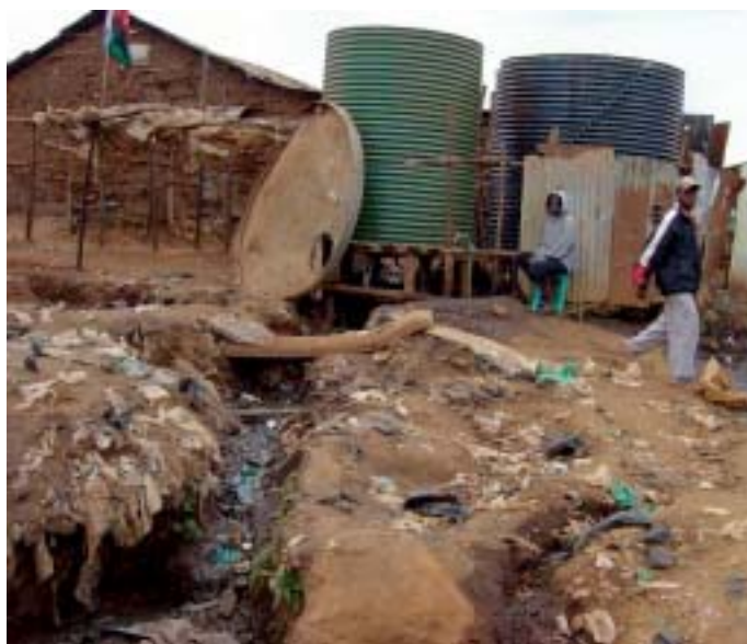
Fig. 2: Water tanks and pit latrines next to a natural run off filled with waste and crossed by a water pipe
