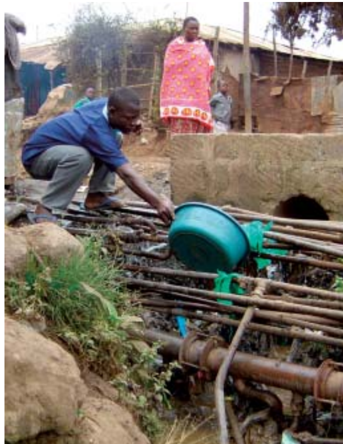
Fig. 3: Man fetching water from a burst pipe
