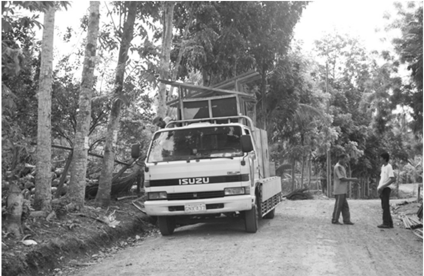
Photo 25: Loading the pre-fabricated udd toilets.
