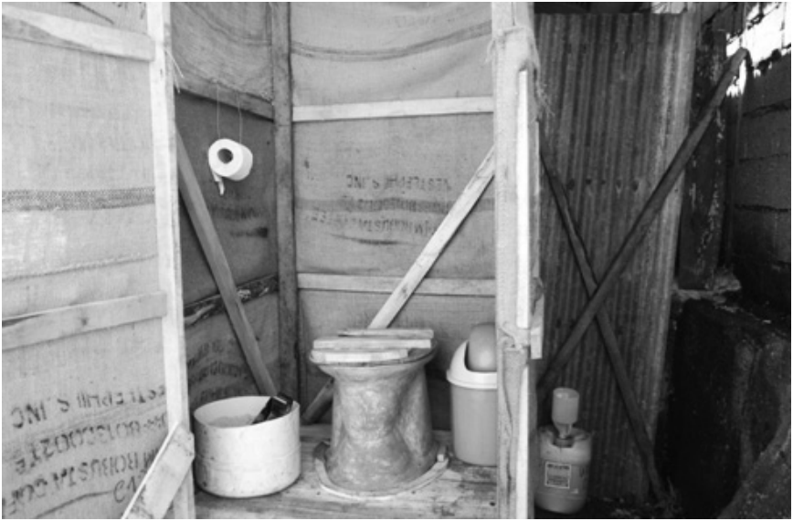
Photo 13: Inside view of a single-vault ecosan toilet. The ash container (white plastic) is at the side while the green container is used for used tissue paper.
