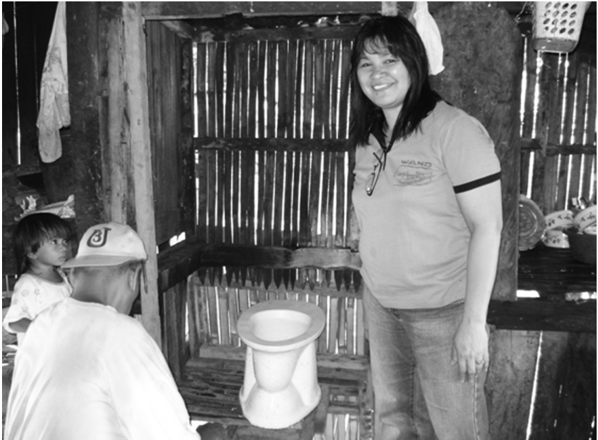
Photo 15: Inside view of a coastal ecosan toilet. The toilet is built at a side of the house that is modified for the purpose.
