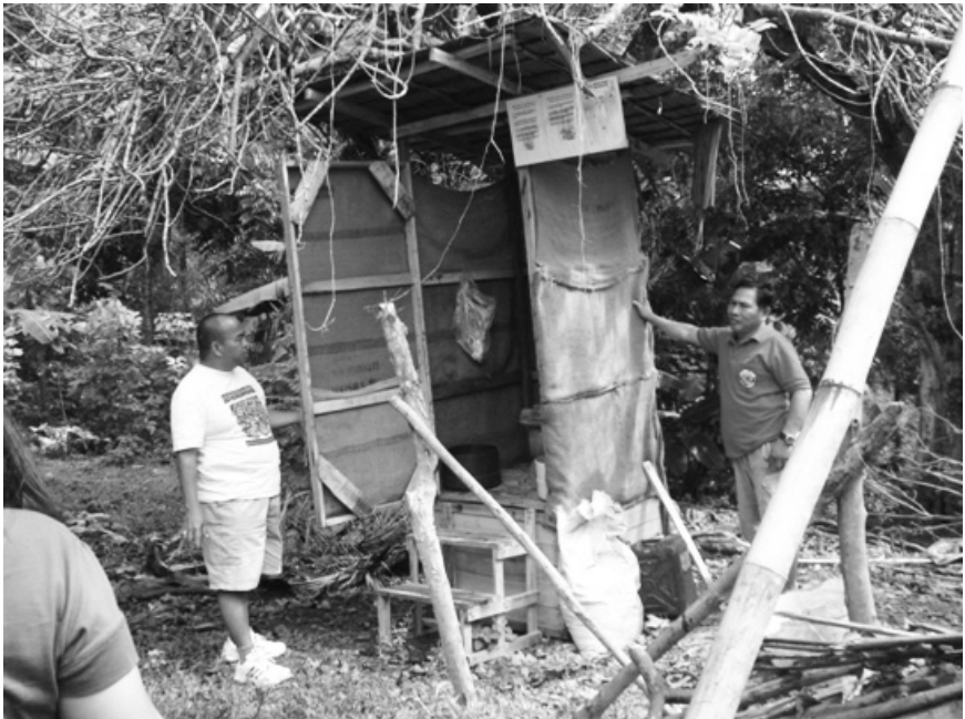
Photo 12: Single-vault ecosan unit using low-cost materials. The frame is made of gmelina wood and coconut lumber, the floor of bamboo, the walls of recycled heavy-duty sacks, the roofing of thatched coconut palm.
