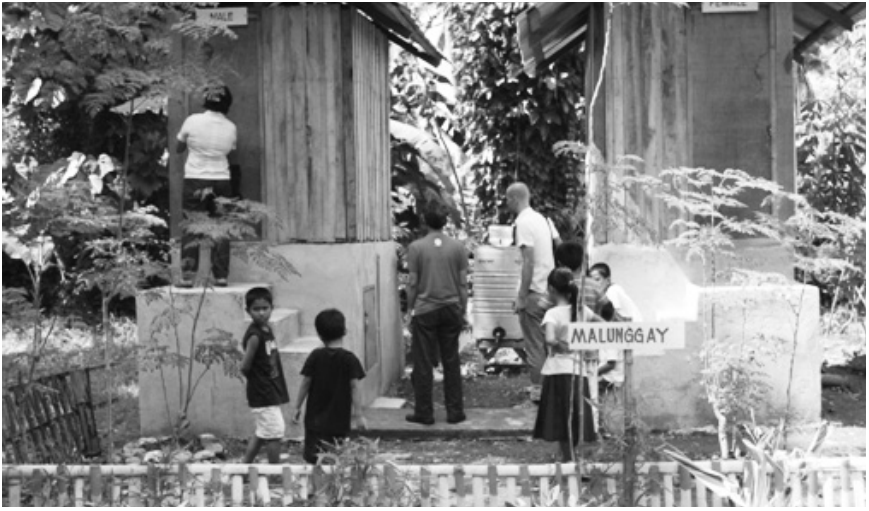
Photo 7: Two double-vault ecosan toilets located in Tuod Elementary School, Manticao, Misamis Oriental. Urine fertilizer is used by the school children in the vegetable and flowers surrounding the school.
