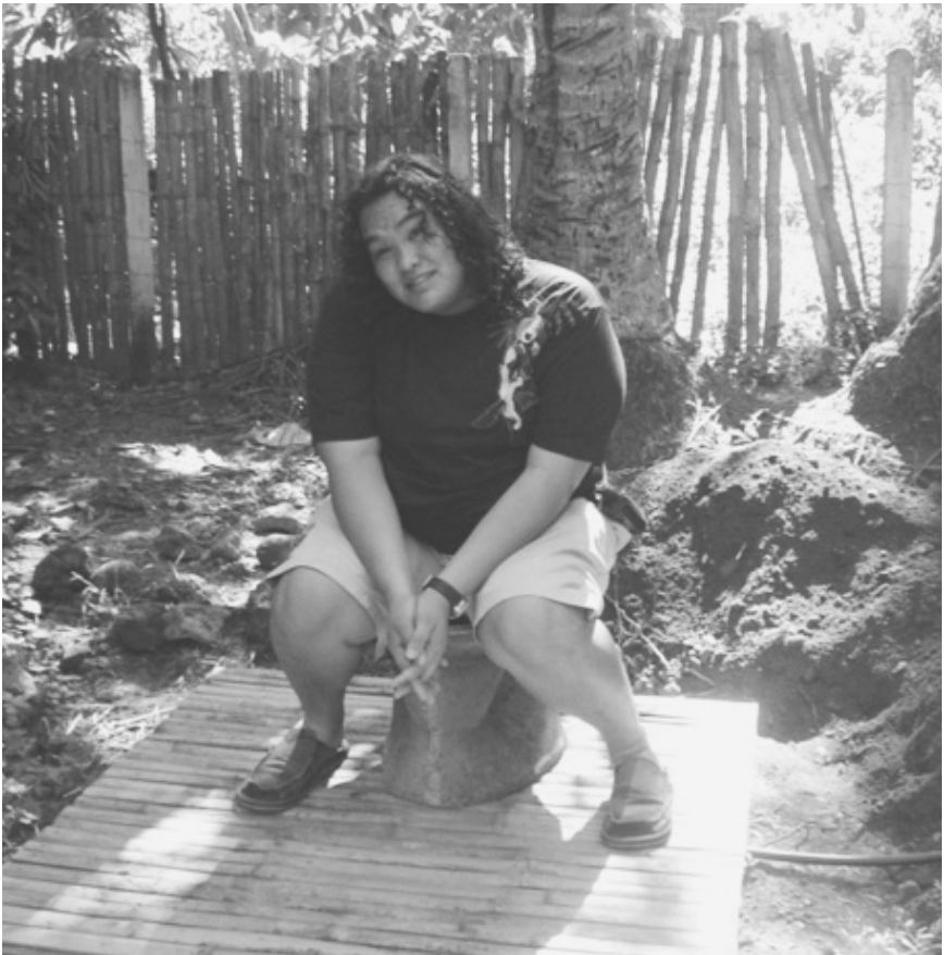
Photo 8: An arborloo cover-slab made of wood poles and bamboo flooring. This is lightweight and appropriate in mountain areas. Two persons or a draft animal can easily carry this. This type of arborloo has urine separation unit.
