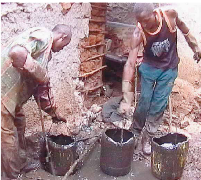
Manual pit emptiers at work, Nairobi (© Sabine Bongsi/WSP)
