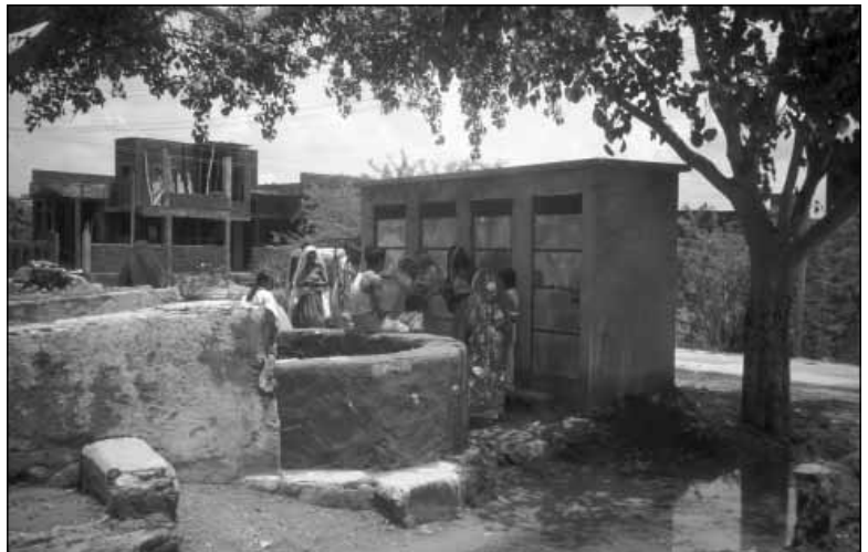
Communal toilet blocks, with women separate from men, are a solution in dense, poor urban areas. Credit: Theo Schilderman, Practical Action
