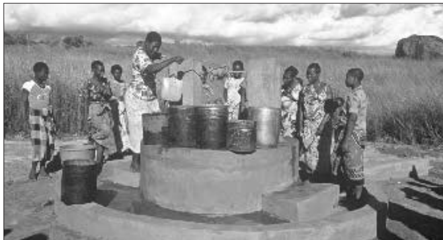
These communities in Niassa Province, Mozambique, chose a protected well with a bucket and windlass because all of the parts could be bought locally and are affordable Credit – WaterAid/Jon Spaul
