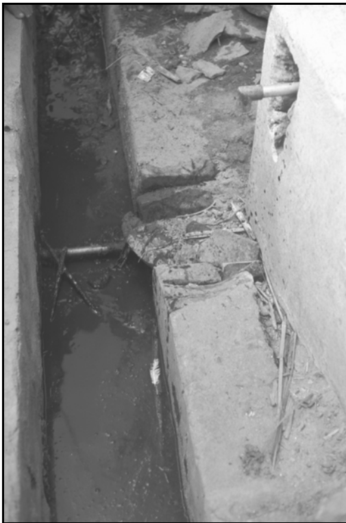
Figure 14: 'Drinking Water' Pipeline Running through a Drainage Canal, Sillamarathupatti
