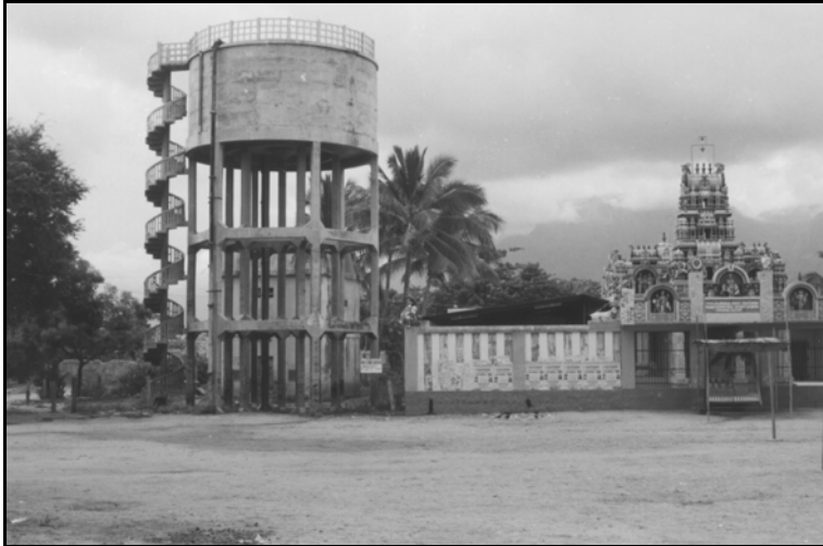
Figure 4: 'Drinking Water' Overhead Tank, Sillamarathupatti
