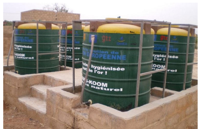
Pic. 4: Tanks with sanitized urine for further distribution as fertilizer in Ouagadougou, Burkina Faso Source: Abdoulaye Fall
