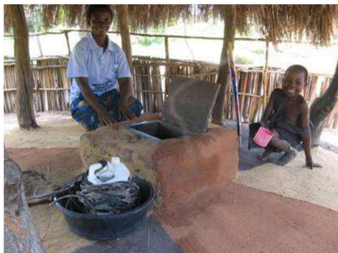
Figure 6 Protected Well in Nchelenge using local materials, and with clean storage of rope and bucket
