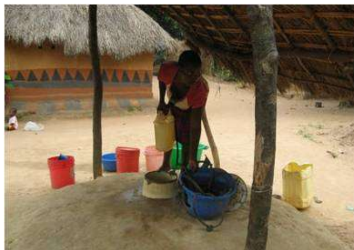
Figure 10 New wells are being constructed with basic elements of protection, starting with the mound, parapet and roof, plus safety of the rope and bucket
