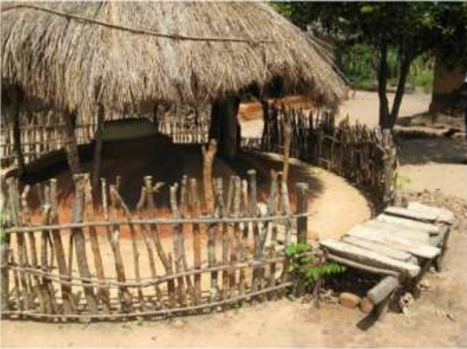
Figure 7 Full set of elements for protection including clay-sealed mound and stand for buckets.
