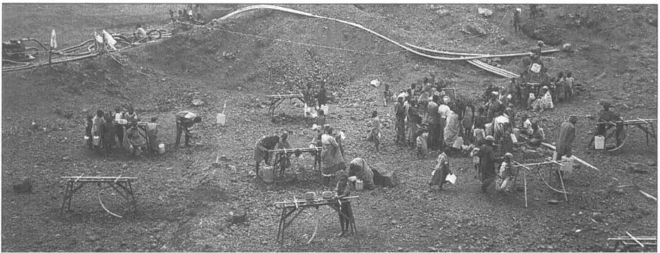
Tapstands being installed and used at Kibumba camp, Goma, September 1994.
