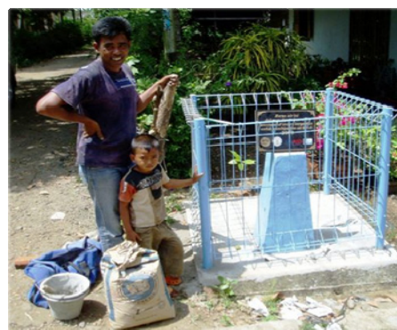
Constructing the Water Spigot Monument, Sukamulya Village, Aceh
